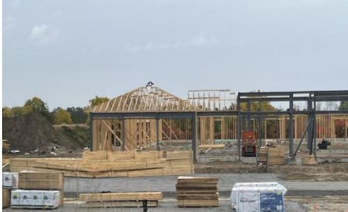
Trusses Installation Begins - Oct. 20, 2025
