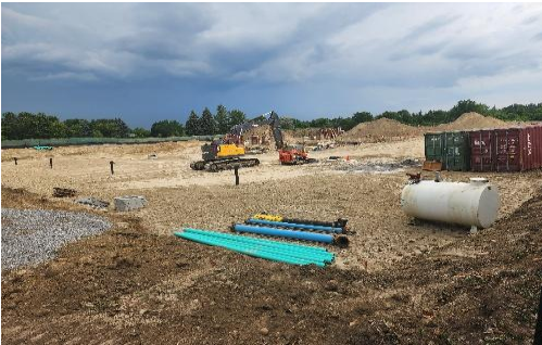
Services Installed – Sept. 22, 2025
