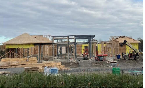
Enclosing the Structure – Nov. 18, 2025
