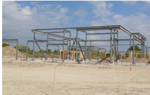
Framing Begins - Oct. 9, 2025
