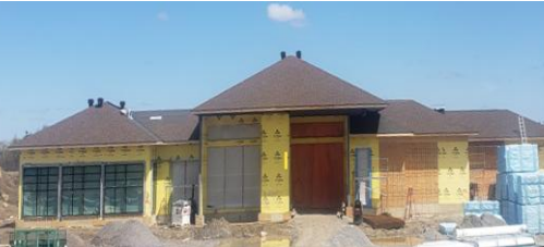
Structure Fully Enclosed – April 16, 2026
